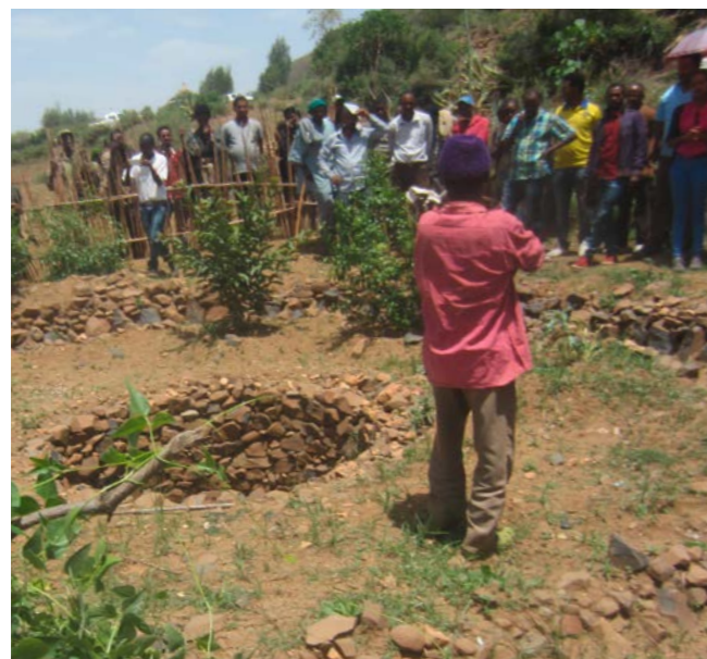
Ring basin infiltration pit (Feb 2016), showing how the intervention functions in severe drought; Gaqiew village, Wag-Himera Zone
